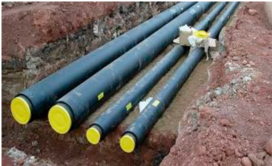
New heating and cooling system
